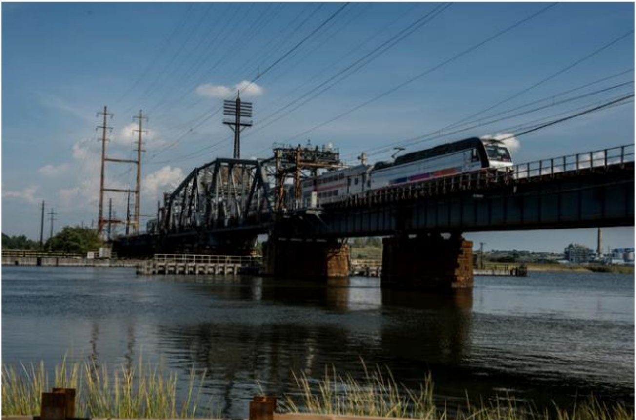
The Portal Bridge, a century-old drawbridge in New Jersey. Officials have the permits to fix it, but without approvals from the Trump administration, construction could be delayed by at least a year.
